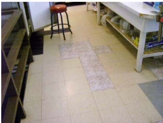
The Kitchen Floor – Old and New Floor
