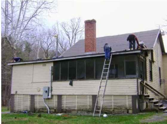
The Dining Hall's New Roof
