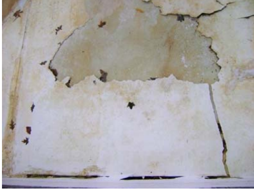
The Swimming Pool Before and During Repairs
